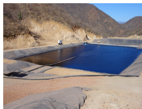
The pregnant leach pond contains copper ions that give it the blue colour of copper sulfate. The liquid is continually pumped to the SX-EW plant. (Courtesy of Red Tiger Mining Inc.)
