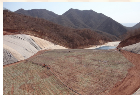
Crushed ore in the leach pad. The pregnant leach pond is in the distance. The crushed ore rests on a leak-proof membrane to protect the underlying ground and prevent the acid and copper ions polluting the local water table.
