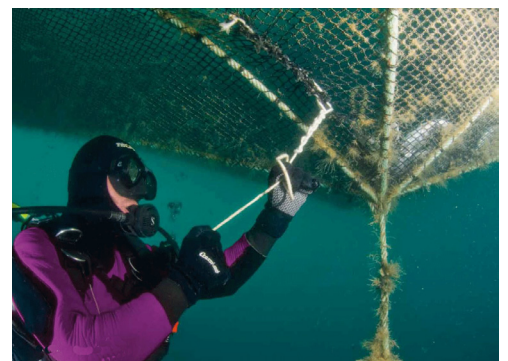
Rope nets can be torn by predators and encourage biofouling. This diver is repairing a tear in the net. (Courtesy of oceanografica.com.)
