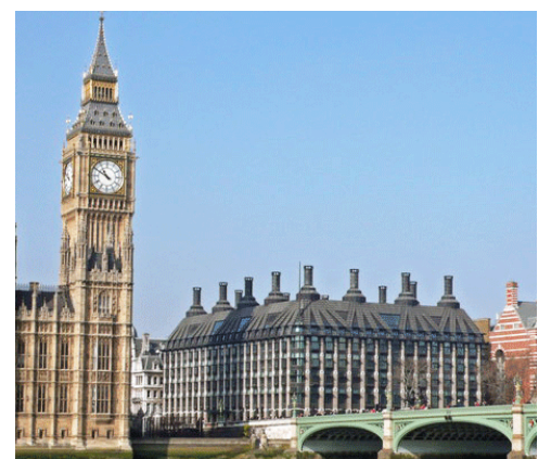
Portcullis House has an aluminium bronze roof and cladding panels. (Creative Commons.)
